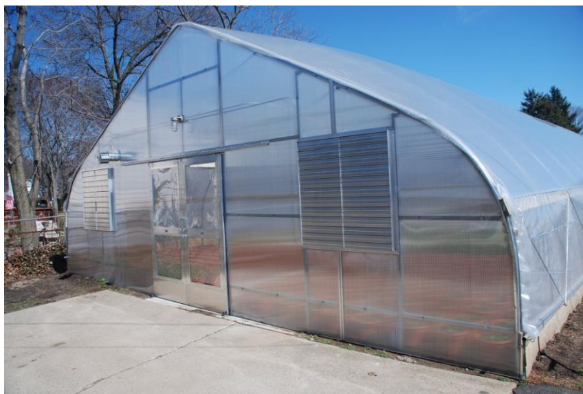
Steel framing. Double sliding doors. Shutters. Polycarbonate
