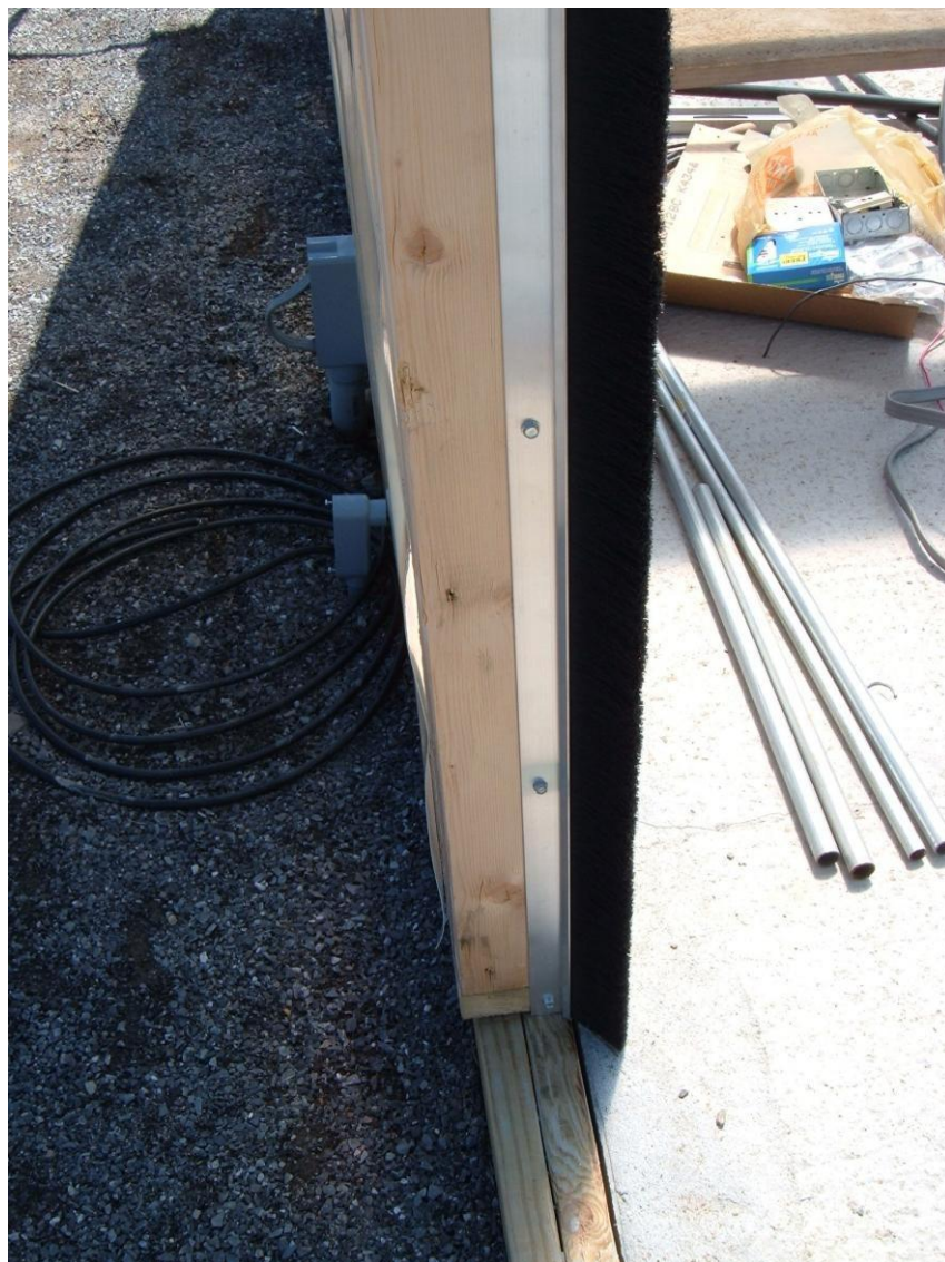
Trac Rite roll up door brush molding. Wood framing.
