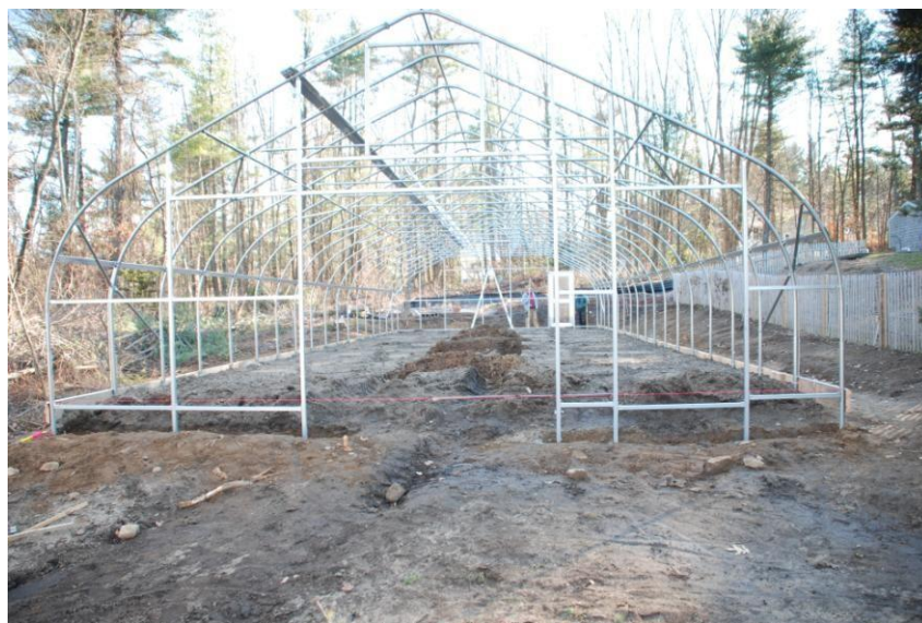
Steel framing. Polycarbonate ends. Roll up door and Plyco door.
