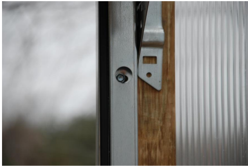
2" tek screw through the Trac Rite fram and wood goes into the steel verticals
