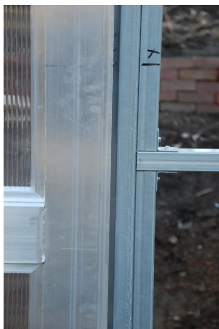
HC pre-hung door with framing doubled up for poly end walls
