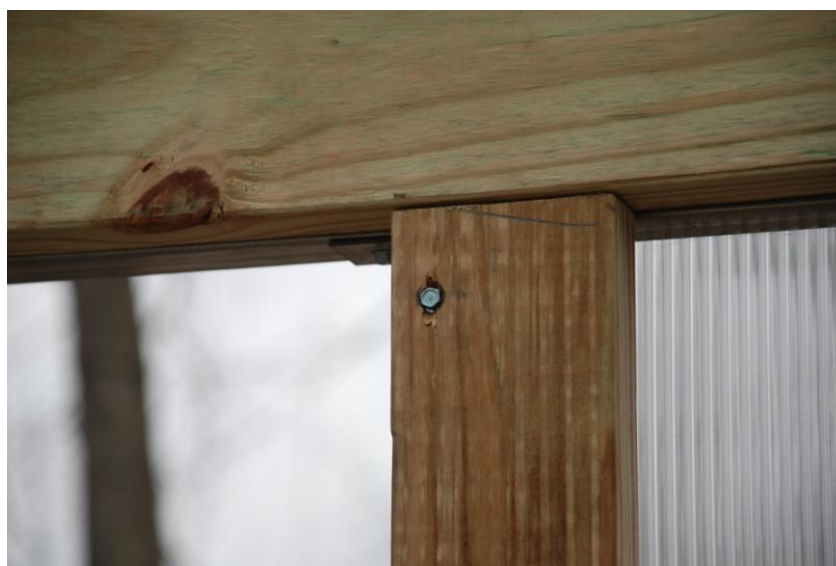
Attach 2 x 4 lumber to the verticals and 2 x 8 lumber for the header using 2" tek screws if the framing is steel.
