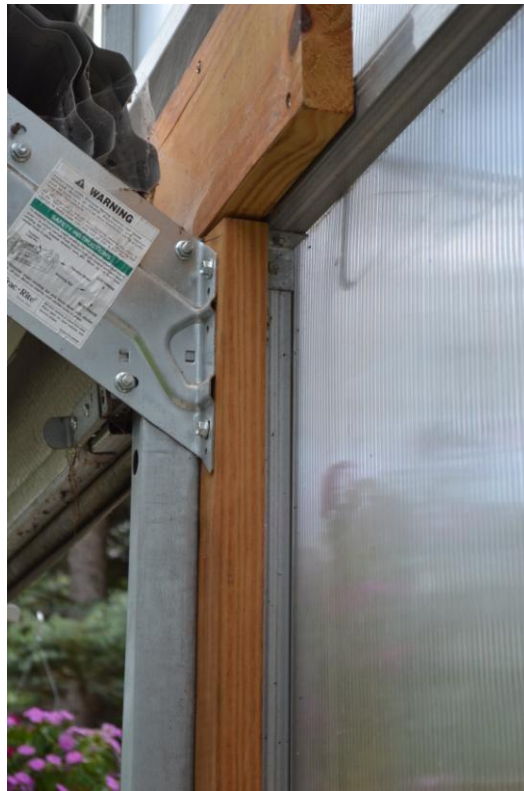
This is what the wood looks like attached to the steel framing
