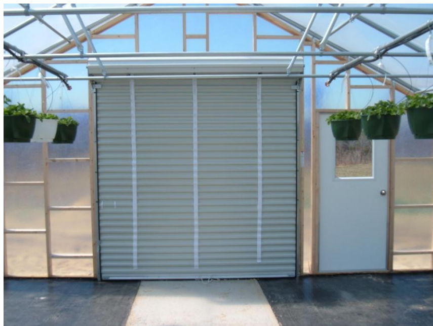
Trac Rite roll up door and Plyco pre-hung door. Wood framing.
