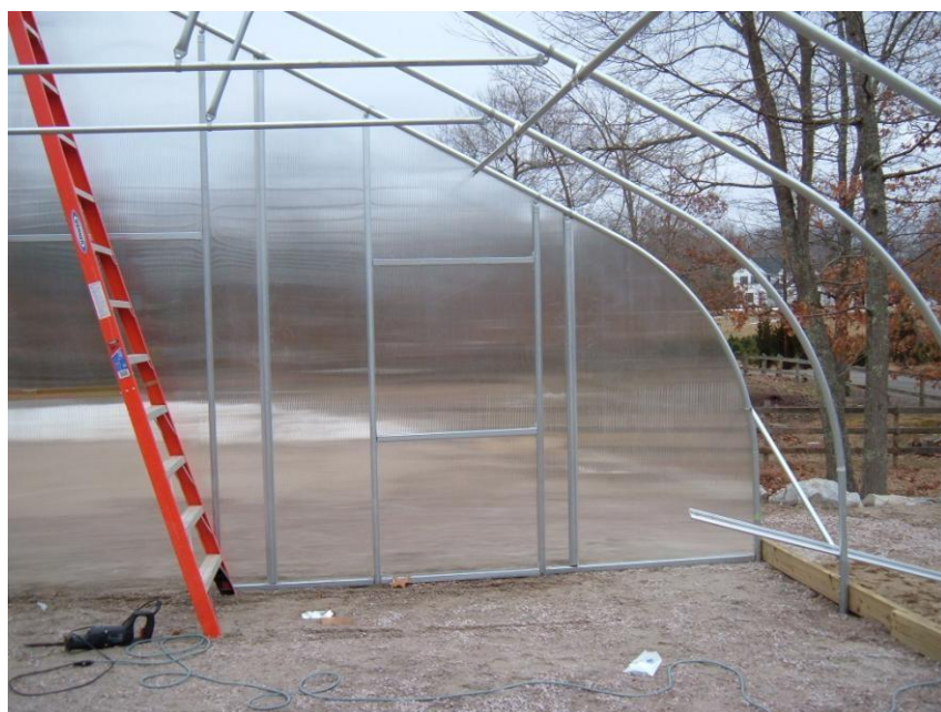
Steel framing. Polycarbonate end wall.
