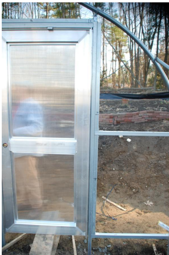
HC pre-hung door with framing doubled up for poly end walls
