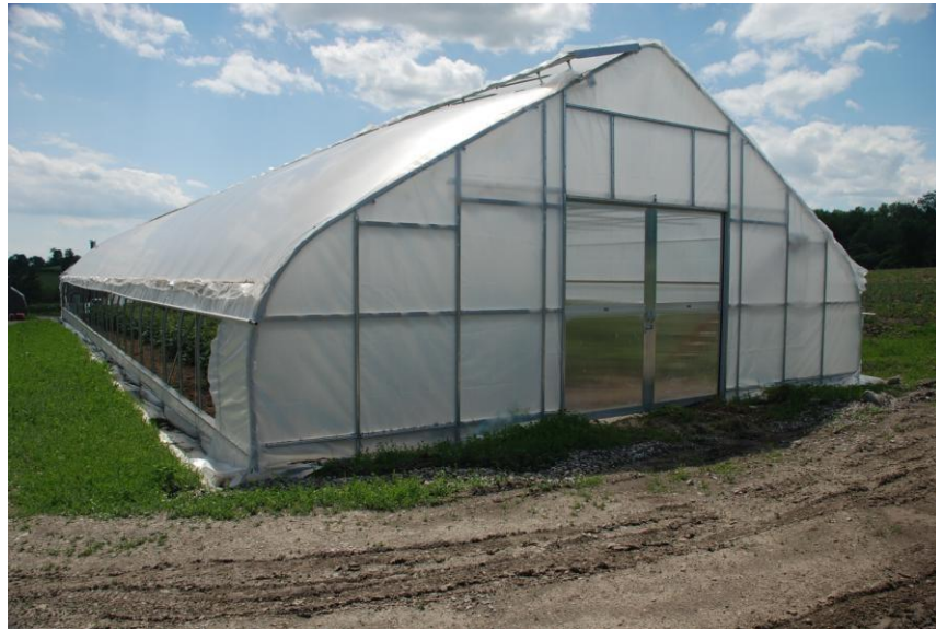
Wood framing. HC double sliding doors. Poly ends.
