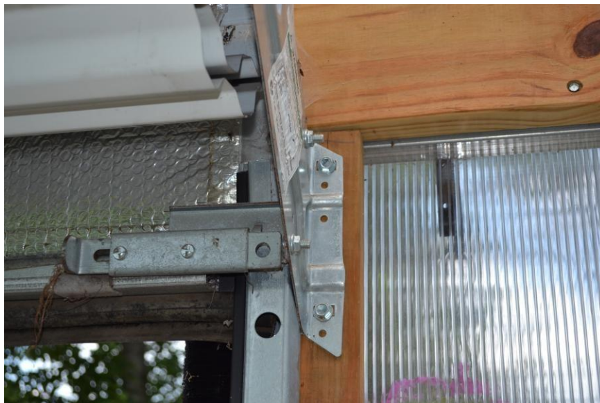
This is how the tabs attach to the wood at the top of the door
