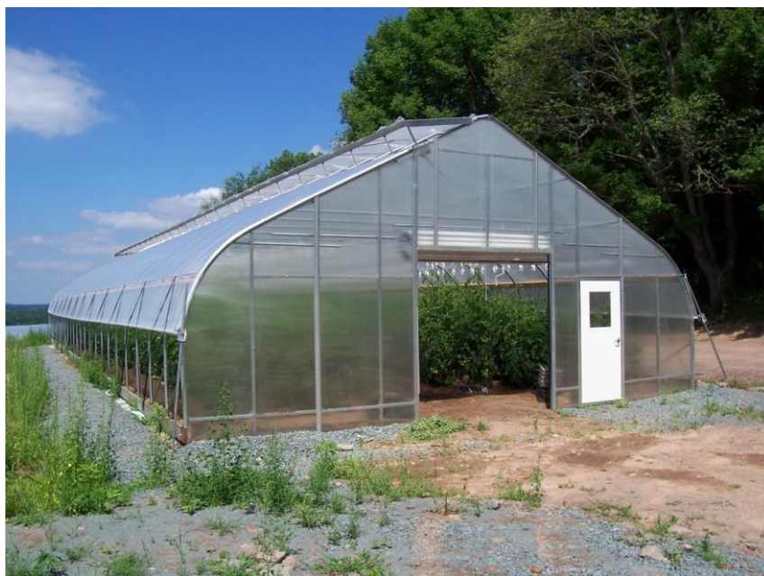
Steel framing. Polycarbonate ends. Roll-Up door. Pre-hung door.
