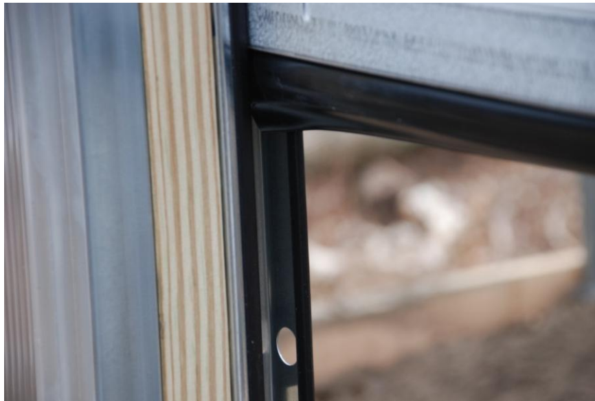
2" tek screw through the Trac Rite fram and wood goes into the steel verticals
