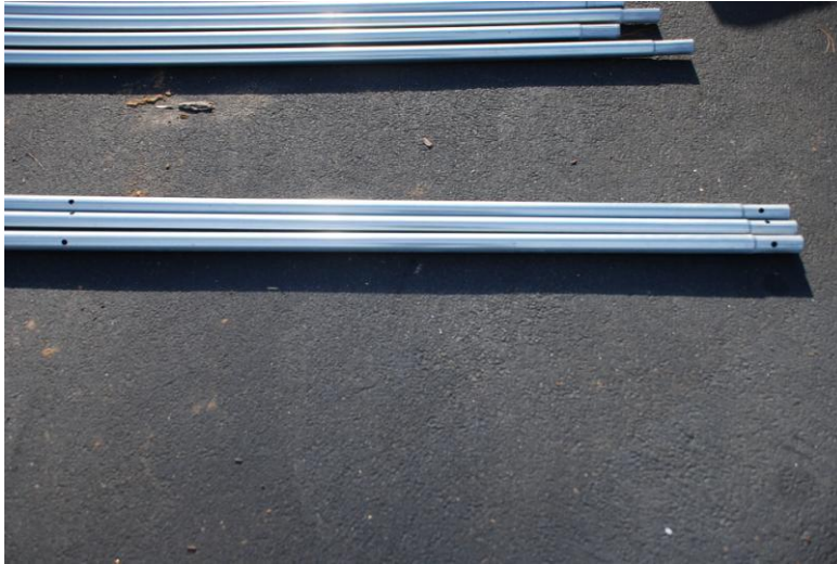
The purlins with holes drilled every 4 ft. are the ridge purlins
