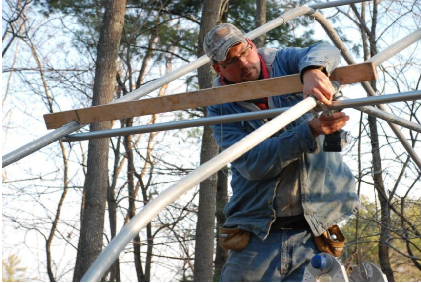
The wooden jig helps line up the bows with the purlin
