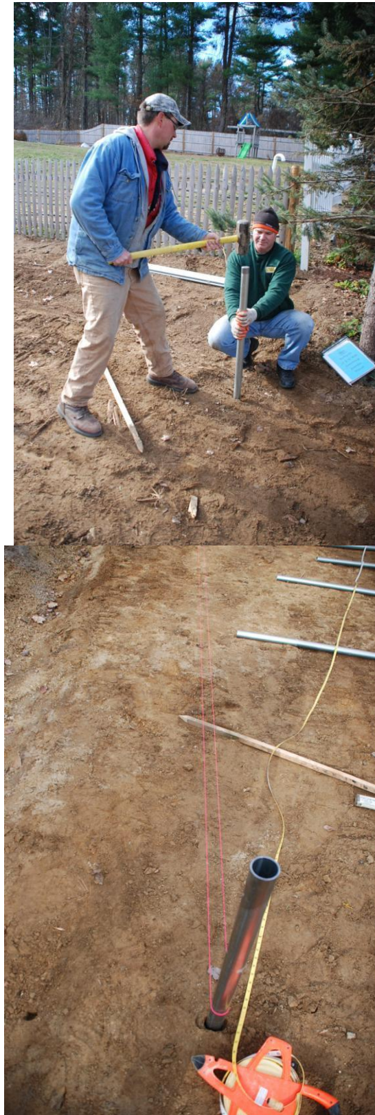
Using a double string wrapped around the end ground posts provides an accurate location for ground post installation
