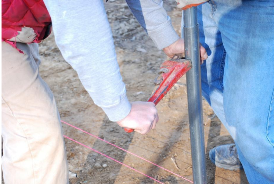
Use a pipe wrench to twist the ground post to line up the holes
